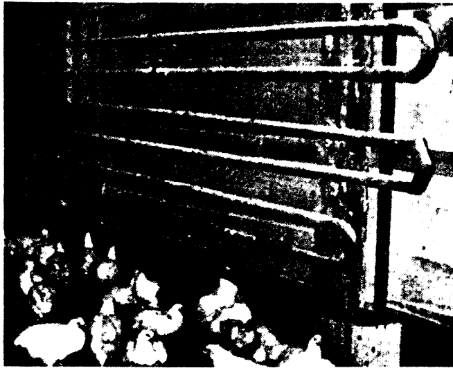
FIGURE 3 HOT WATER PIPES HUNG ON THE WALL
